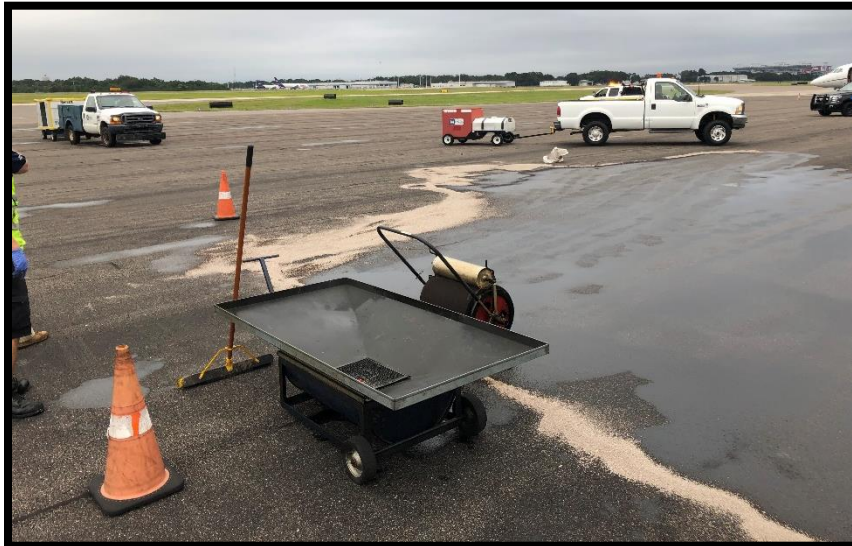
Granule absorbent material can be difficult to remove from a scene.
