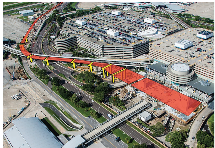
The Airport will close the roadways in front of Blue Arrivals and Departures to allow for steel beams, some weighing as much as 146,000 pounds, to be placed into position on the SkyConnect Guideway. The project will go on until early 2017, with breaks during high traffic periods, including holidays.
