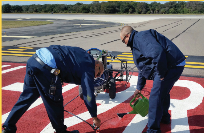
Maintenance employees Alex Rivera (left) and Mike Mitchell (right) repaint the airfield markings to exact specifications following the rubber removal project.
