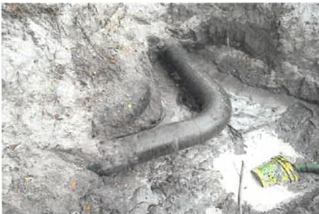
12-inch Piping View
