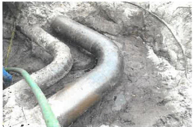
18-inch Piping View
