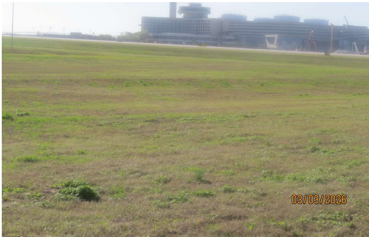
Looking southeast across the Northwest RON Apron project area from the edge of Taxiway V.
