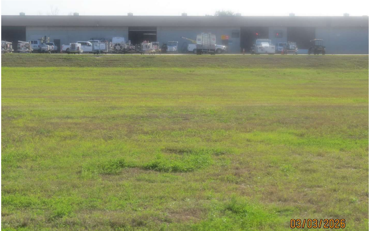
Looking east across the Northwest RON Apron project area toward the North Cargo Facility from the edge of Taxiway V.
