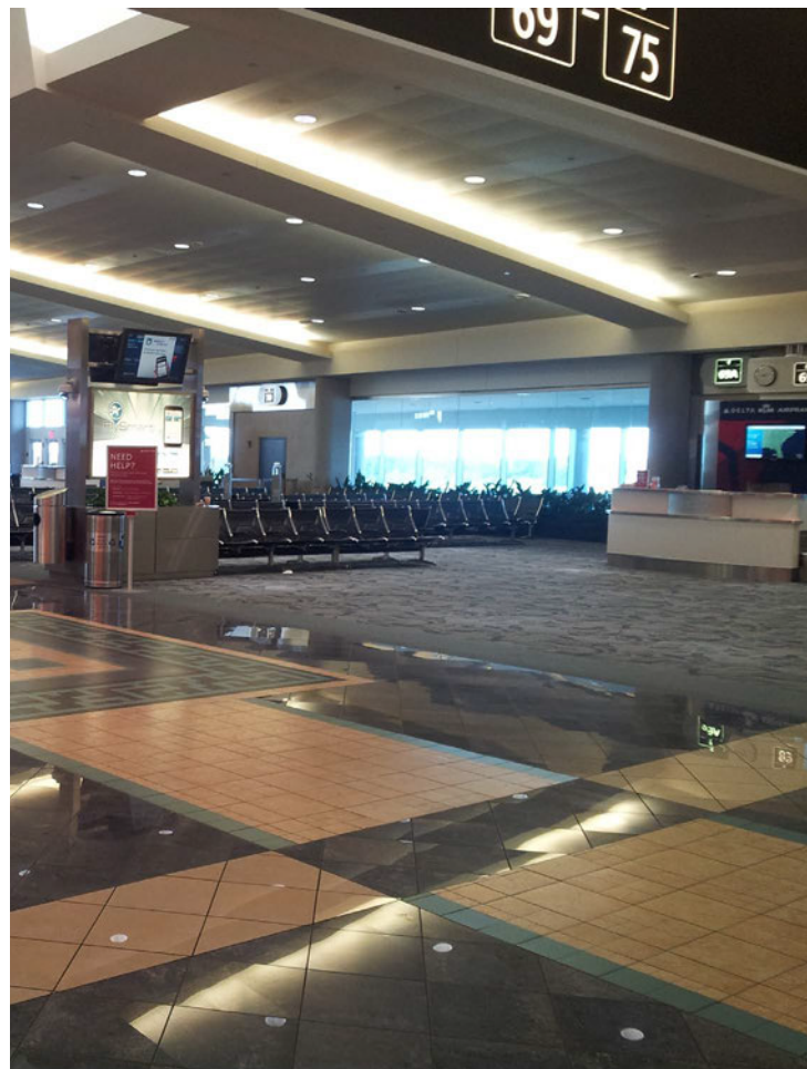
Central zone looking southwest: This is a typical ceiling condition where the ceilings align with the column bays forming room size zones for each gate lounge.
