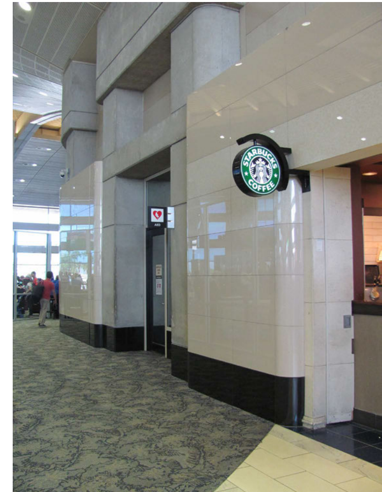
Typical concourse fixed element façade: Polished soft neutral porcelain ceramic panels. These hold the space and yield much freedom for concessionaire insertions to be colorful, textural and saturated.
