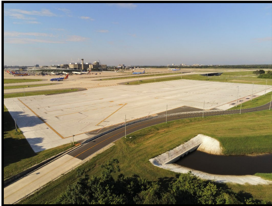
North RON Hardstand
