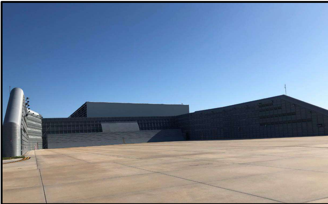
The Maintenance Run-up Enclosure is also commonly referred to as The Hush-House.
