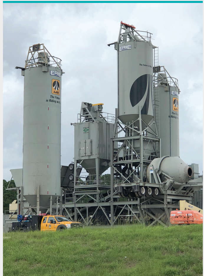
The concrete plant helps reduce travel time and cost.
