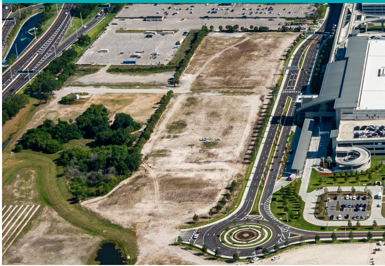
Crews are already performing enabling work on the empty lot shown here.
