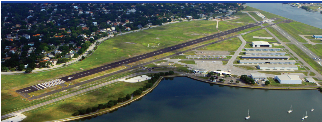
Tampa Bay General Aviation airports have a combined $87 million impact per year.
