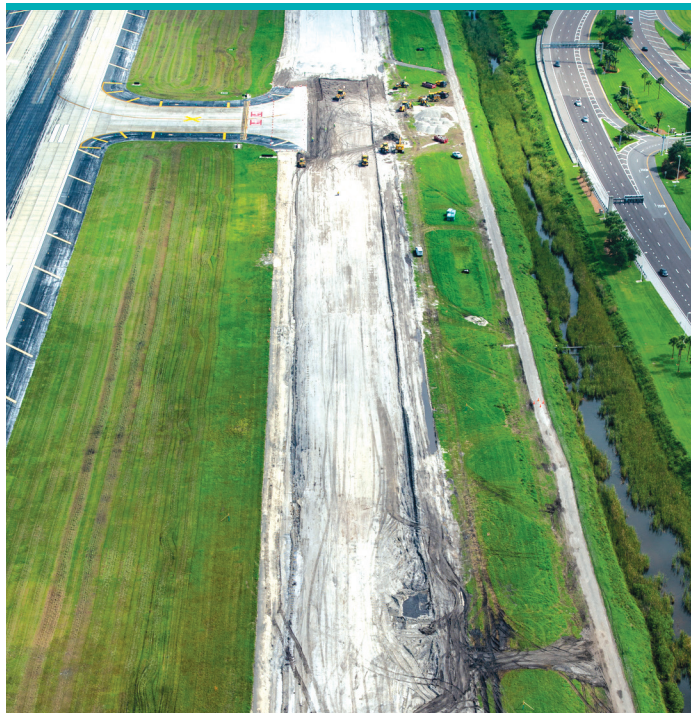
Crews are upgrading Taxiway W, pictured in this recent aerial photo by Aerial Innovations. In total, they'll redo 5,000 feet of taxiway.
