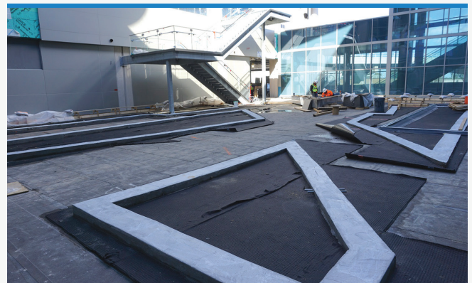
Crews are currently building two outdoor courtyards, including the northeast courtyard pictured above. The space will be a quiet place to relax.
