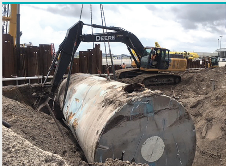
Construction crews remove one of the five 20,000 gallon storage tanks.
