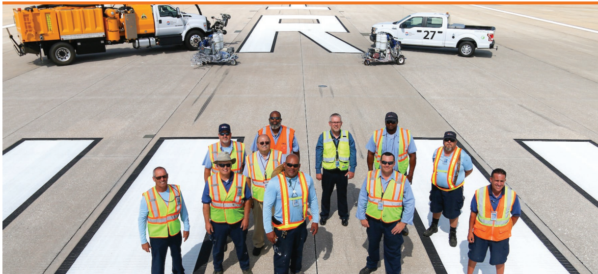
The TPA airfield team completed the largest in-house airfield maintenance project in TPA's history in February.
