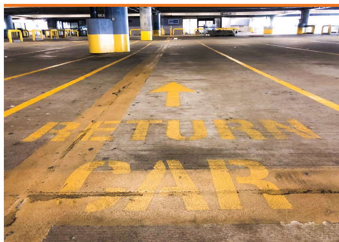
Crews are beginning to reclaim the first two levels of the Long Term Garage. The first new level could be open in six months.
