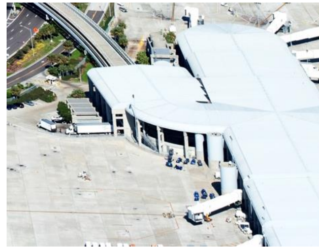
Large Structural Columns
