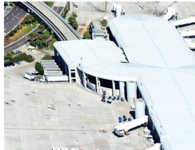
Large Structural Columns
