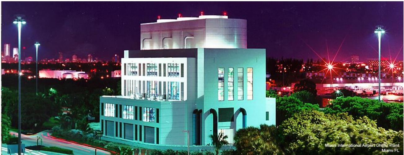
Miami International Airport Central Energy Plant
